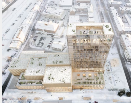
▲ Sara Kulturhus a 20-storey building mainly constructed from locally sourced wood, creating both an architectural landmark and an example of advanced timber engineering. Designed by White Arkitekter. © White Arkitekter
