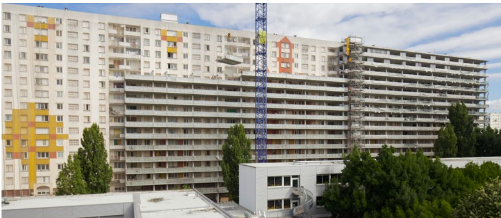
◀ Transformation of 530 dwellings, Grand Parc Bordeaux, France, 2017. (case study 25) Architects Anne Lacaton, Jean-Philippe Vassal, Frédéric Druot, Christophe Hutin. Winner of the 2019 EU Mies Award. © Philippe Ruault
