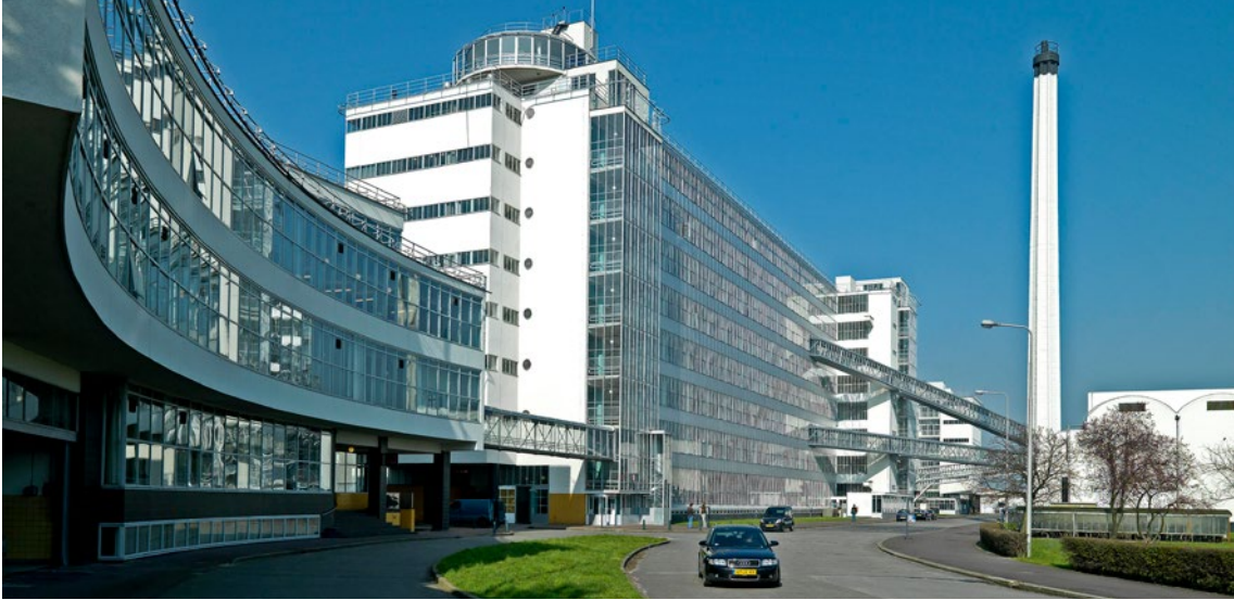
▲ Van Nelle Factory, Rotterdam, Netherlands. Designed by Leendert van der Vlugt, renovated by Wessel de Jonge. Winner of the 2008 European Heritage Award, conservation category. Courtesy of Europa Nostra
